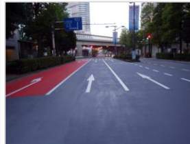
Toshima Ward Tokyo Thermal barrier pavement
